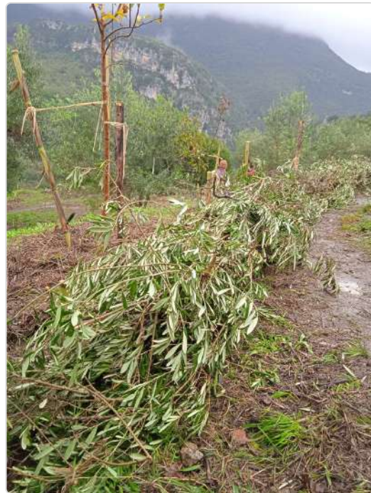
Bio-rolls example at the end of the first terrace.
